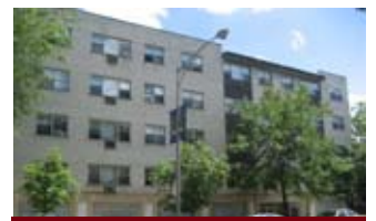
Tuscon Apartments Sheridan Road Offering Chicago, IL
